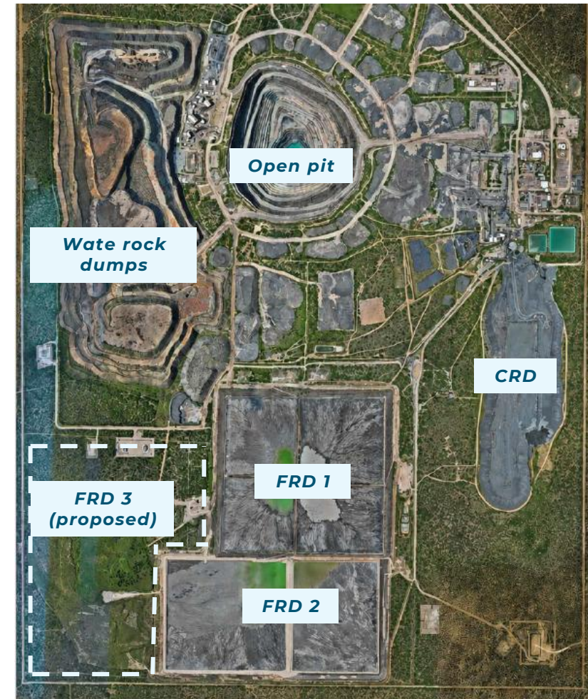
Aerial view of Karowe Tailings Facilities
